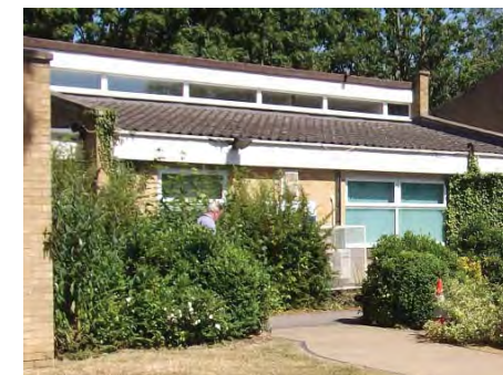
Figure 4.7 Health centre, Exeter Close
